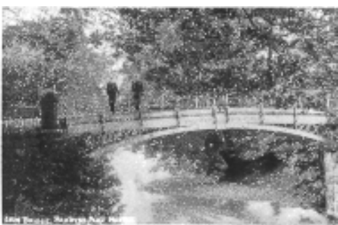
The 1813 Iron Bridge in Brabyns Park.
